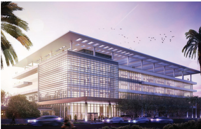
UHealth Lennar Foundation Medical Center
