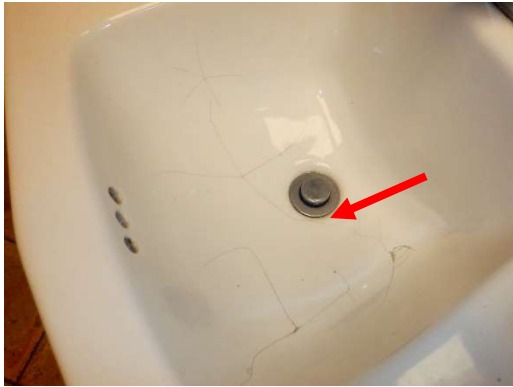
Cracked Bathroom Sink
