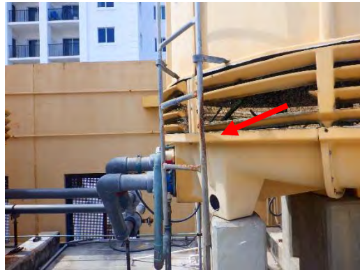
Corroded Ladder
