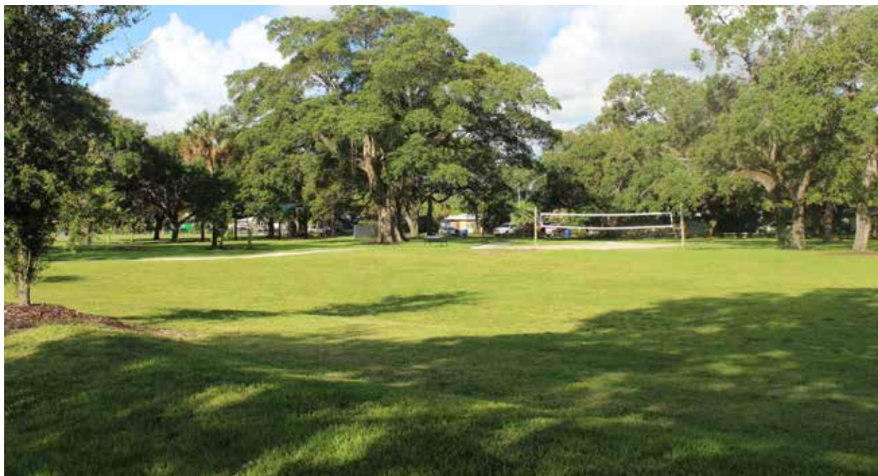
Hott Park, Fort Lauderdale- Sunken multi-purpose field used as detention basin during severe storm events
